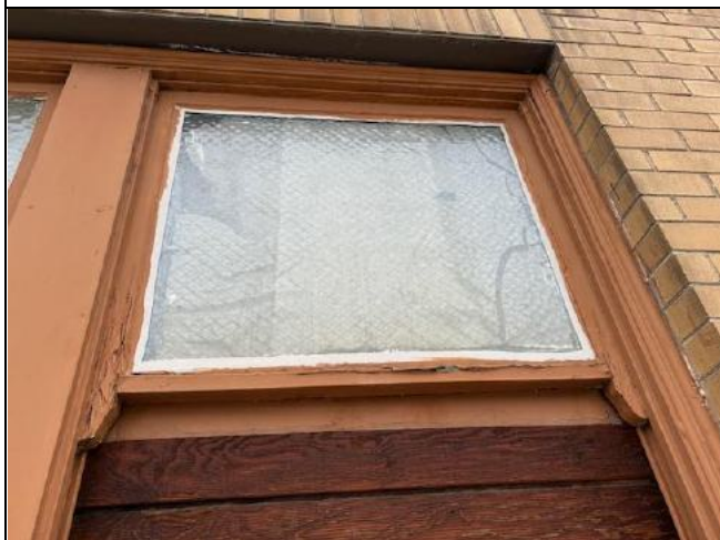
View of Window Glazing – Brown/Gray Window Glazing (ACM) Located on the South Exterior Roof. (Photograph 5)
