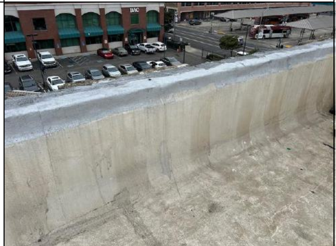
View of Silver Roof Coating – Black Roofing Material (ACM) Located on the Roof Parapet. (Photograph 4)
