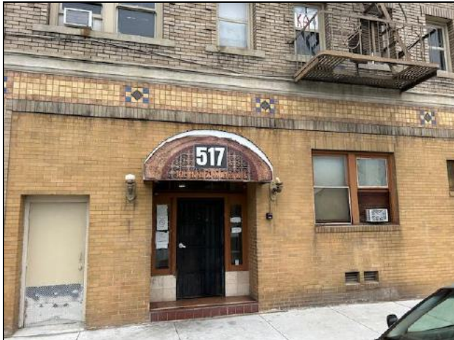
View of Building Exterior – 517 Channel Street, Stockton, CA. (Photograph 1)
