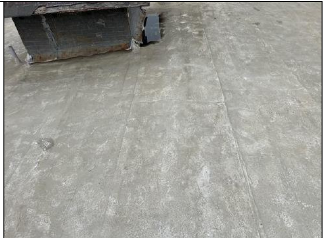
View of Rolled Roofing with White Coating (ACM) Located on the Roof. (Photograph 2)
