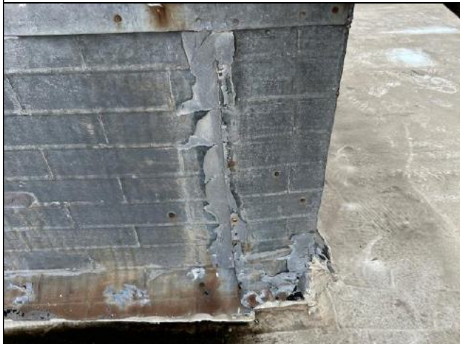
View of Gray Roof Mastic (ACM) Located on the Roof Vent. (Photograph 3)
